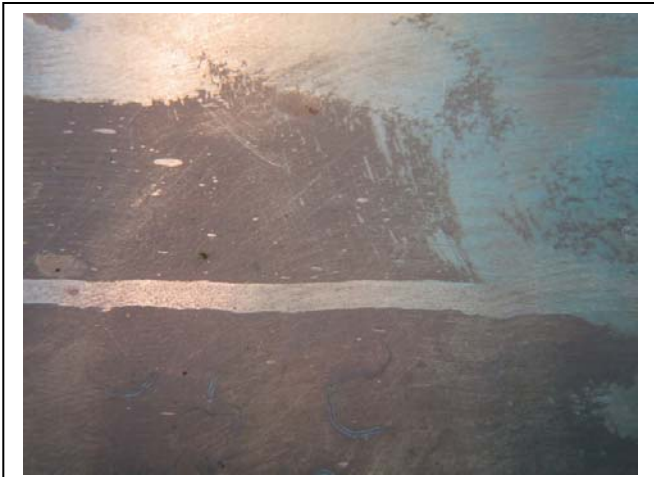
Some areas near the .4 radius appeared to have been missed during the coating process; these uncoated areas were approximately two grades rougher than the coated surfaces.
