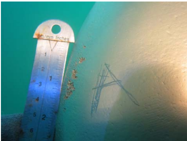
Blade A: Cavitation on .9 radius 2.5 inches in length. Surfaces around the cavitation damage appeared to still have intact coating.
