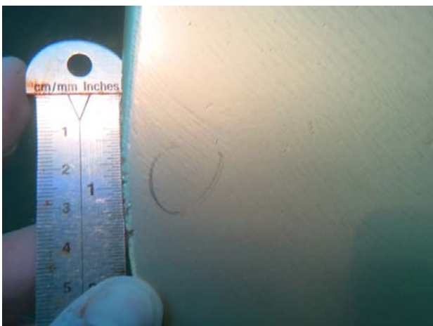
Blade C: Cavitation at the .9 radius, 1.5 inches in length. Surfaces around the cavitation damage appeared to still have intact coating.
