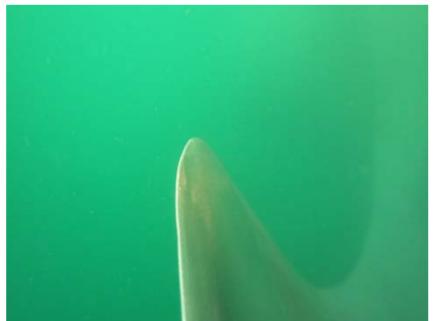
Blade F: fouled with light slime on leading and trailing edge. Tube worms were observed on the pressure face and suction back. Coating in good condition overall.
