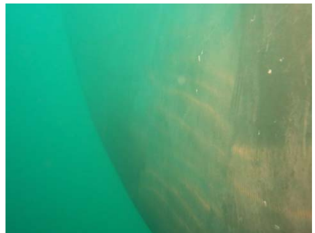
Blade E: fouled with light slime on leading and trailing edge. Tube worms were observed on the pressure face and suction back. Coating in good condition overall.
