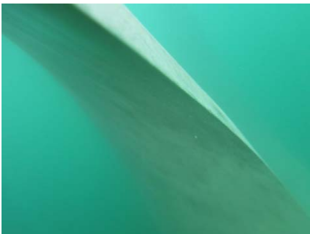
Blade C: fouled with light slime on leading and trailing edge. Tube worms were observed on the pressure face and suction back. Coating in good condition overall.
