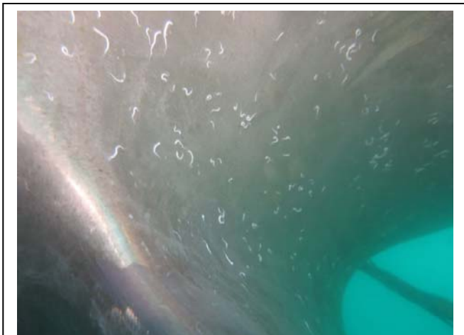
Blade A: fouled with light slime on leading and trailing edge. Tube worms were observed on the pressure face and suction back. Coating in good condition overall.
